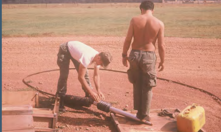
DaNang Air Field: Chaffin is the guy with his hands greasy installing rubber donuts on an arresting cable. During an arrestment, it was common for these donuts to be ripped from the cable.
